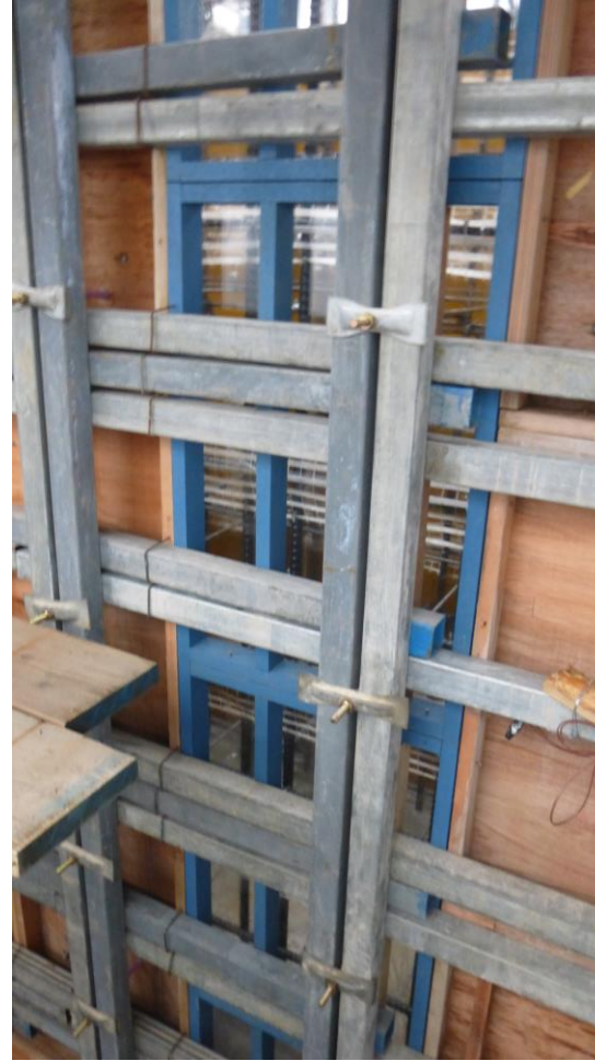
透明樹脂製型枠 (青枠)
